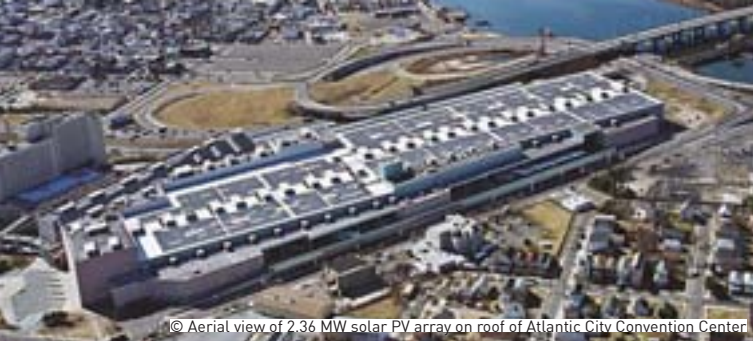
© Aerial view of 2.36 MW solar PV array on roof of Atlantic City Convention Center
