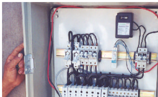
A custom-made AC electricity meter of high sensibility has been employed in order to measure low energy consumptions.
