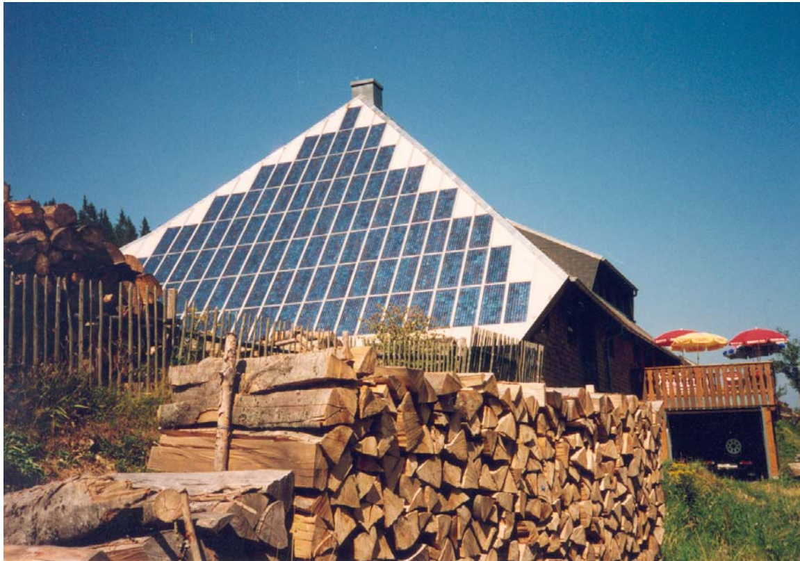
Fig. 3: First solar powered inn - the »Rappenecker Hof«. A PEM fuel cell will be added to supplement and – in the long range – to replace the diesel generator in the this hybrid system. Planning is ongoing, begin of operation of revised system design including the fuel cell is 3 rd quarter of 2003.
